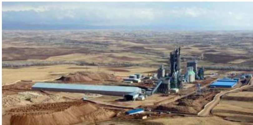
Figure 9. Shahrak iron ore concentrate Plant
