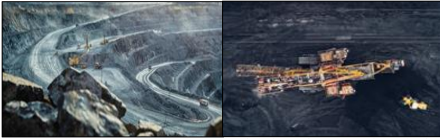
Figure 1. Hunter valley, New South Wales, an aerial view of an open pit coal mine, Australia ( https://www.shutterstock.com , 2024)
